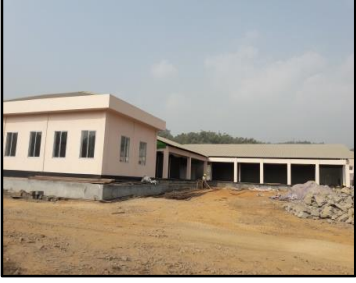
CONSTRUCTION OF MARKET
