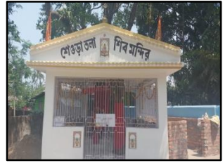
PUBLIC UTILITY AREA AT GOURI KOUN
