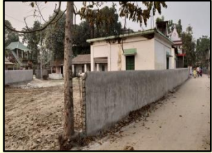
BOUNDARY WALL CONSTRUCTION
