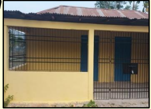
SCHOOL BUILDING RENOVATION
