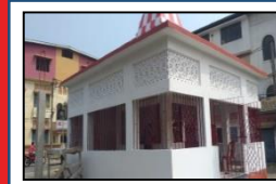
PUBLIC UTILITY AREA
