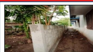
BOUNDARY WALL CONSTRUCTION
