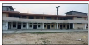
CLASS ROOM CONSTRUCTION
