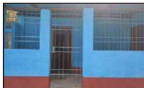
SCHOOL BUILDING RENOVATION
