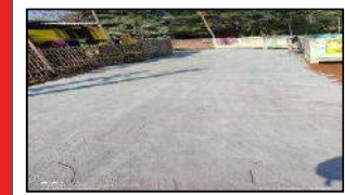
CONSTRUCTION OF RCC ROAD
