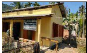
SCHOOL BUILDING RENOVATION
