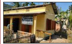
PUBLIC UTILITY AREA CONSTRUCTION
