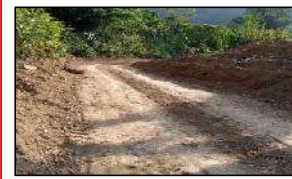
PUBLIC UTILITY AREA CONSTRUCTION
