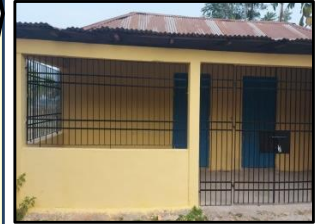
SCHOOL BUILDING RENOVATION
