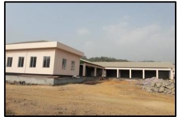
CONSTRUCTION OF MARKET
