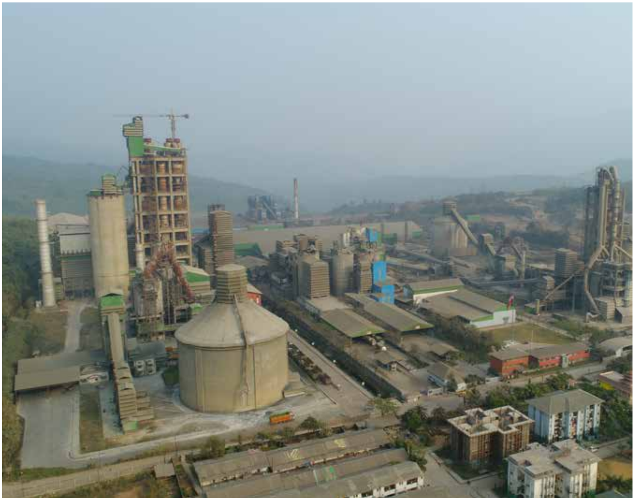
Aerial view of Star Cement plant in Meghalaya.
